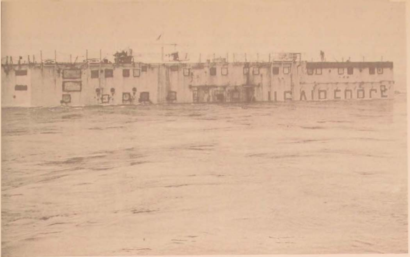
A helicopter lands crewmen on the 1600-ton structure as it is towed to Kearny, New Jersey. Its lower deck is welded shut and filled with urethane foam for flotation.
