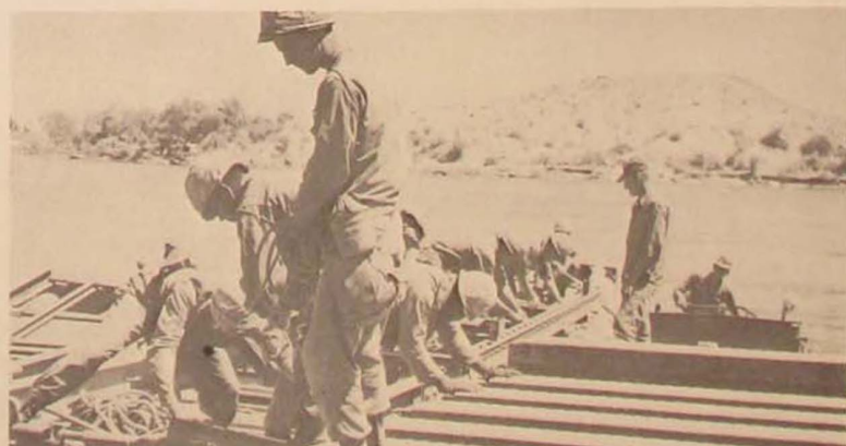
Army engineers lift pontoons into the Colorado River. . . . The bridge company fits raft sections over pontoons before laying the trackage for tanks.
