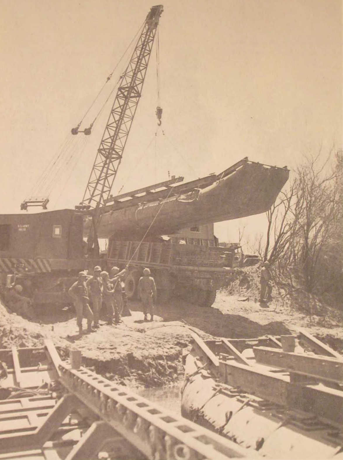
Army engineers lift pontoons into the Colorado River. . . . The bridge company fits raft sections over pontoons before laying the trackage for tanks.
