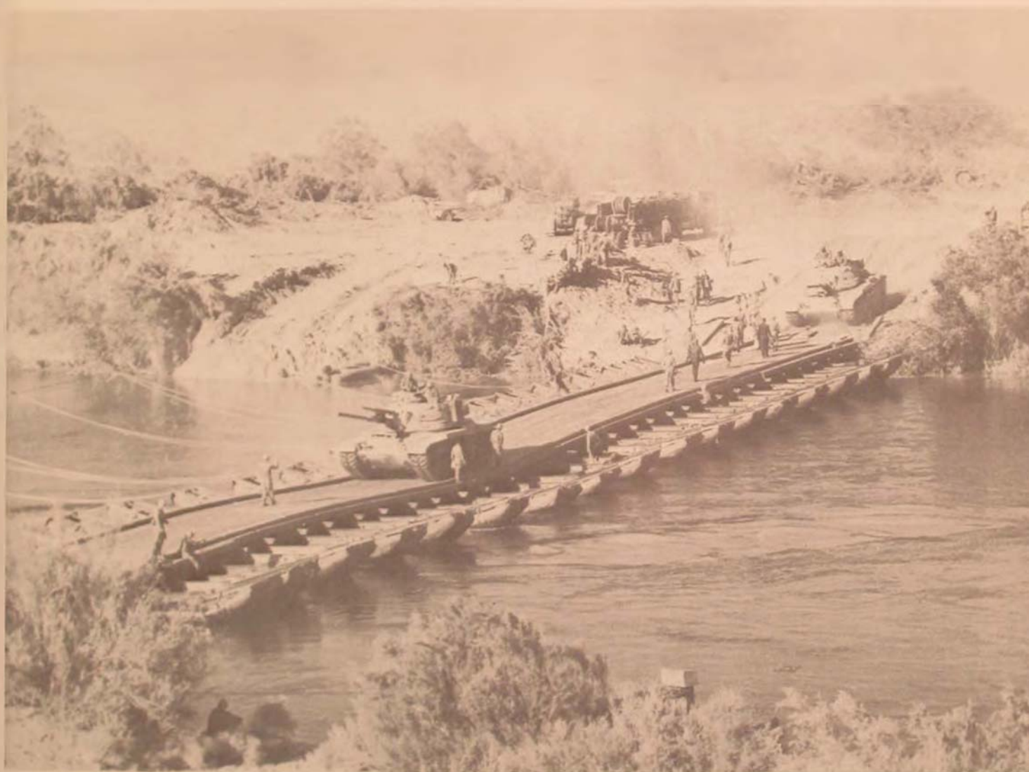
Pontoon bridge construction proceeds from both sides toward the middle. . . . M-60 main battle tanks of the 2d Armored Division are first across the newly completed floating pontoon bridge.
