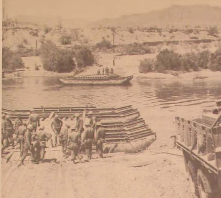
Pontoon bridge construction proceeds from both sides toward the middle. . . . M-60 main battle tanks of the 2d Armored Division are first across the newly completed floating pontoon bridge.
